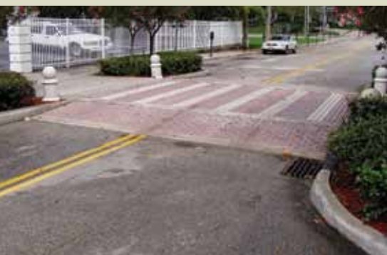
SOURCE: WWW.PEDBIKEIMAGES.ORG/DAN BURDEN
