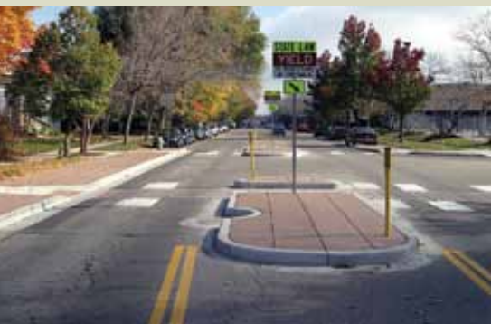
SOURCE: WWW.PEDBIKEIMAGES.ORG/DAN BURDEN
